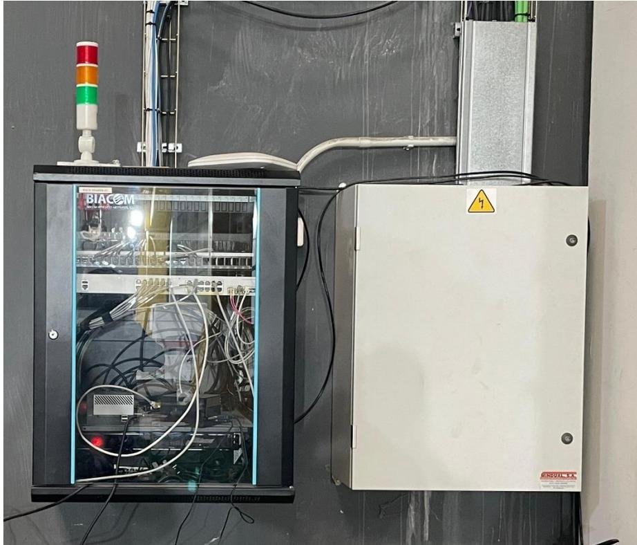
*Figure 9: Fibre optic cabinet. Electric cabinet.*
